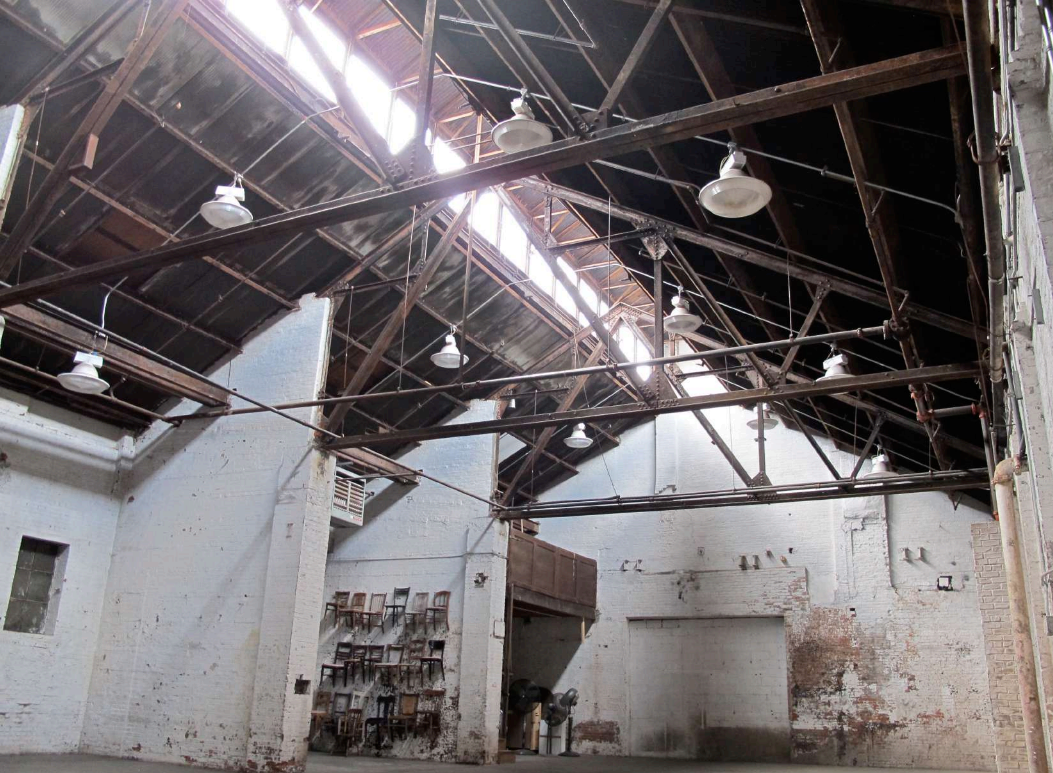
Area 3: West Wall
