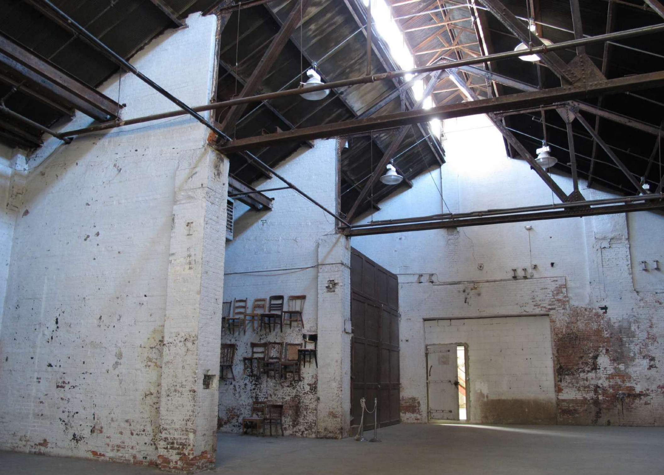
Area 3: West Wall with Door to Area 4
