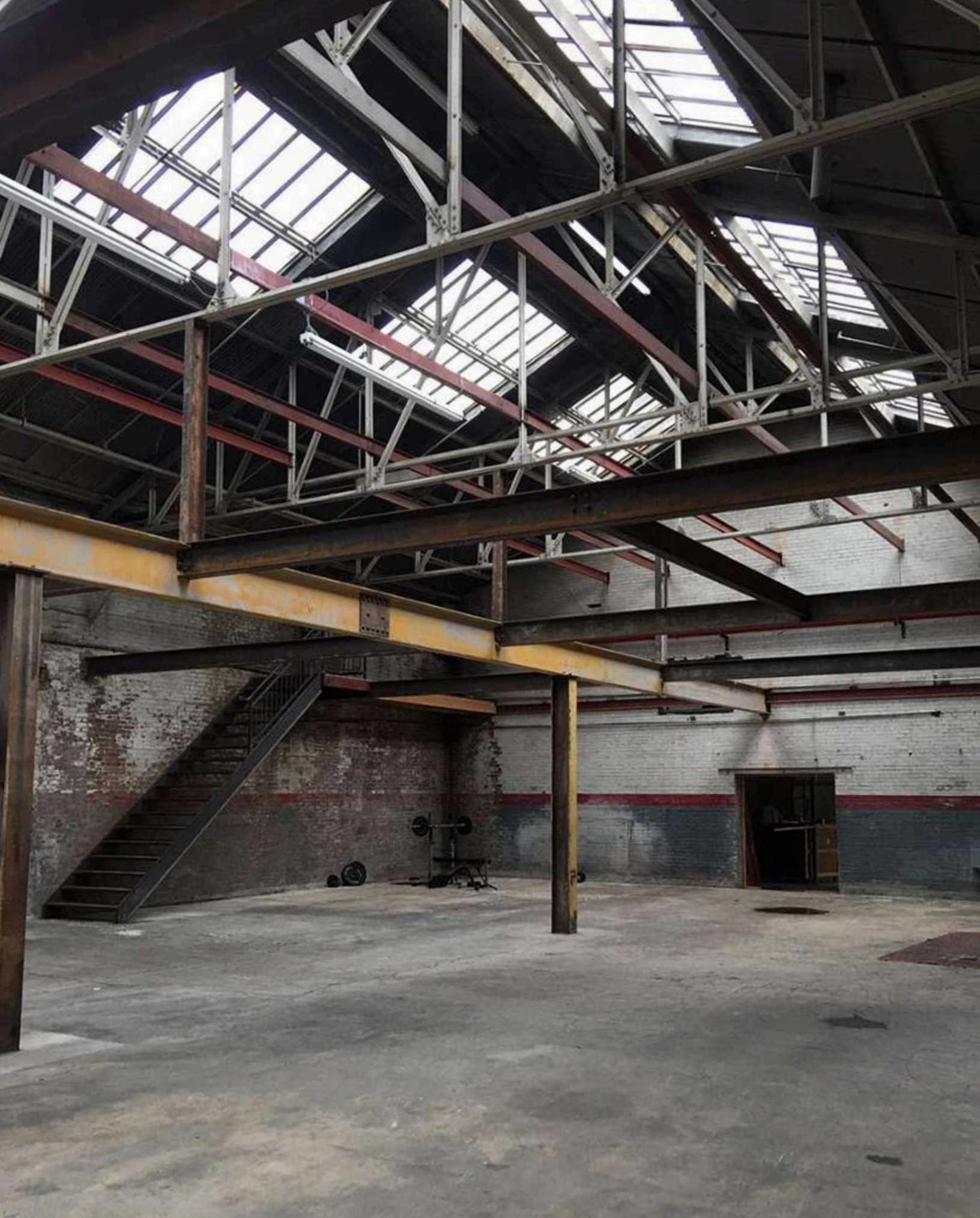
Area 5: North East Corner, Double Doors to Area 4
